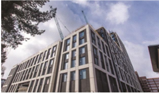
Brick faced sandwich panel with fair faced concrete finish
