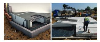
Spantherm is a high performance off-site concrete flooring system. A typical plot can be installed in just 90 minutes, cutting up to a week off the schedule.
