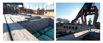
Homespan is a rapid build system and intallation is completed in under 2 hours for a typical house type. Installation is unaffected by weather which reduces labour time on-site.
