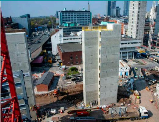
Rapidcore lift and stair cores are manufactured offsite in bespoke moulds and are installed quickly and efficiently by our specialist installation teams. Creagh can design and manufacture the capping slabs with all temporary and permanent anchors cast in. Rapidcore can also be designed as shear walls to provide lateral stability or as an efficient replacement for blockwork or in situ concrete.
