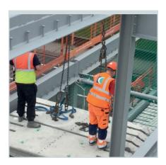
The installation of precast planks will be carried out by trained precast installers under the supervision of a lift supervisor and SSSTS qualified supervisor. Once the lifters are attached, additional safety chains are placed around the plank for safety of installation.
