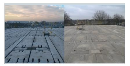
Tie bars and grouting will be carried out by a wet works team. Ready-mix grout will arrive to site and concrete pumps will be used. A banksman will be used to assist with the positioning of the concrete pump. Where grout is mixed on site this will be carried out by an operative wearing FFP3 dust masks who have been facefit tested.
