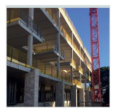
All open edges will have a propriety edge protection system or scaffolding erected to provide edge protection.
