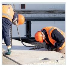
The slinging of the units will only be carried out by a trained CPCS trained slinger/signaller. The slinger will ensure that the load is secure and safety chains are fitted to the precast floor units correctly prior to carrying out the lift.
