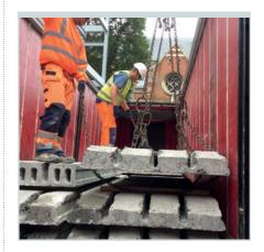
All chains and lifting equipment will be visually inspected and recorded on a LOLER. This document will be completed weekly. Chains will have a visual inspection each time they are used, checking for damage from buckling or frayed slings. If the chains or slings are damaged they are discarded and marked -
