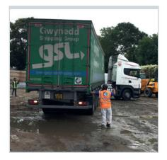
On arrival to site, the delivery vehicle will be met by a Creagh banksman and banked into position for unloading, as per the lift plan.
