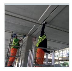
Finishing works will be carried out by fully trained operatives using scaffold or podiums, while grinding operatives will wear impact goggles, ear defenders, FFP3 dust masks and trained face fit personnel.
